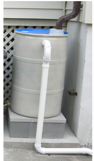
Rain barrel captures runoff.
