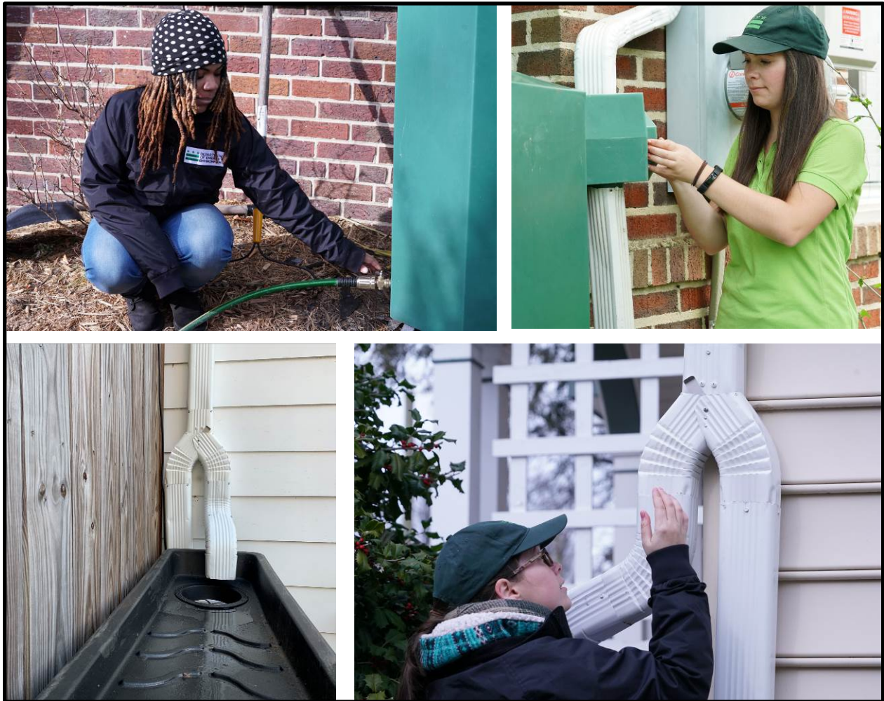
Series of photos depicting barrel maintenance. Top left: closing the spigot in the spring. Top right: cleaning the filter sock on the diverter box. Bottom left: cleaning the top and filter basket. Bottom right: adjusting the y-diverter toggle for the spring.
