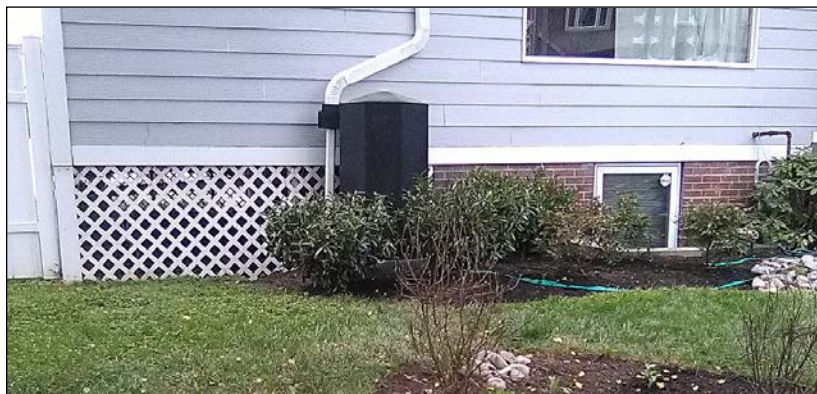
Barrel attached to a rain garden
